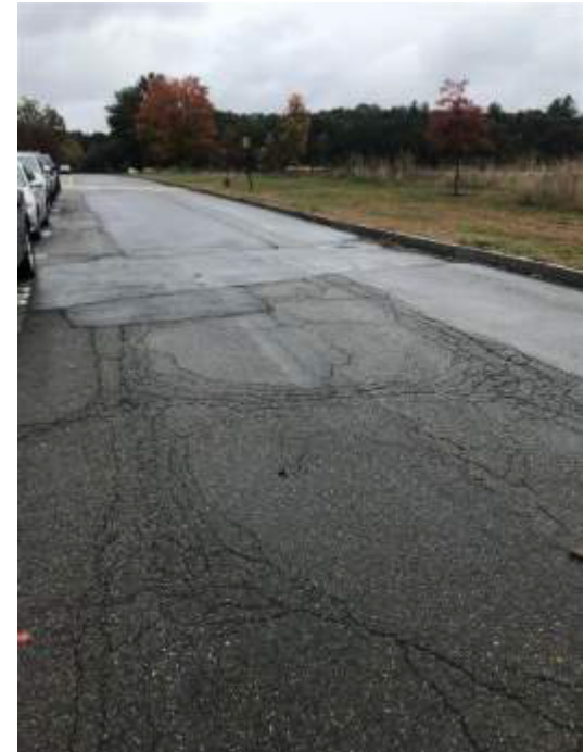
Multiple patches and significant cracking
