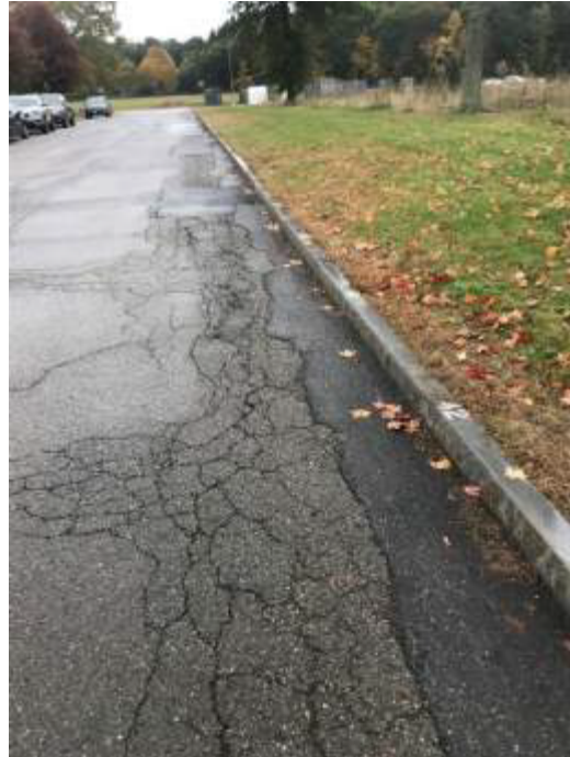
Multiple patches and significant cracking
