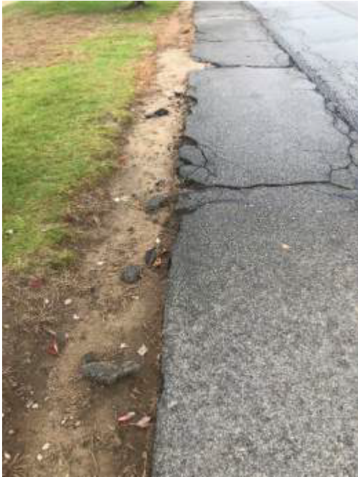
Broken and spalled pavement on sidewalks
