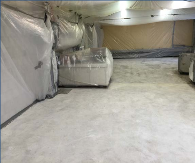
Ripley Copy Center Asbestos Flooring Replacement
