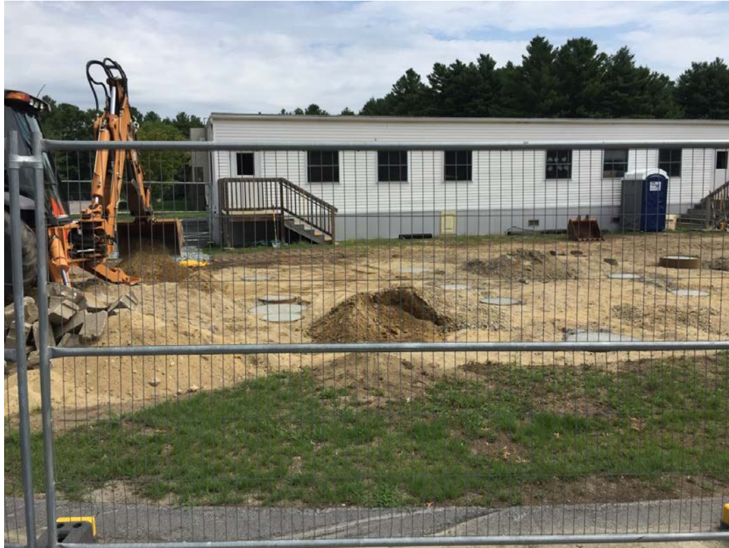
Sanborn Modular Classrooms Installed
